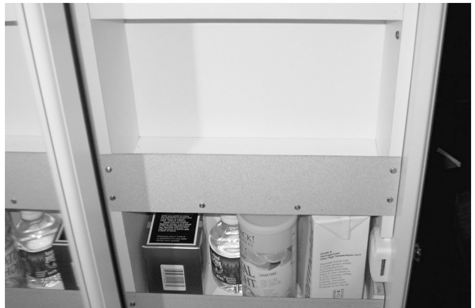
Strips of plastic laminate replace the railings on pantry shelves, allowing for the storage of larger items in the pantry
