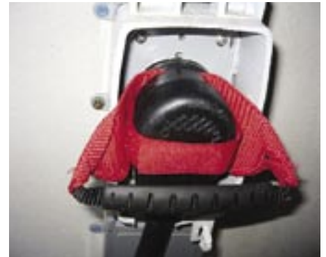
Plug dog makes disconnecting easier.
